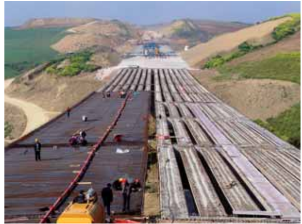
East-west motorway/western section Autouroute Est-Ouest / Lot Ouest Autopista Este-Oeste/Tramo Oeste
